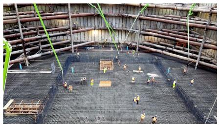
**Concrete Placed at Bottom of Excavated Shaft**
