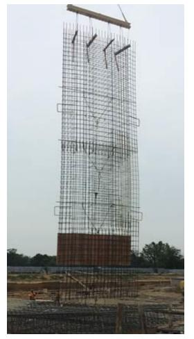
Insert Steel Reinforcing Cage and Place Concrete
