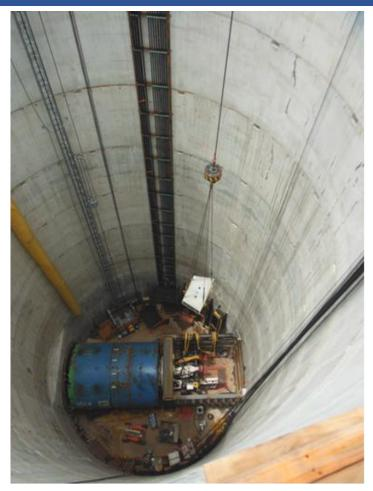
**Tunnel Boring Machine in Tunnel at Bottom of Shaft**
