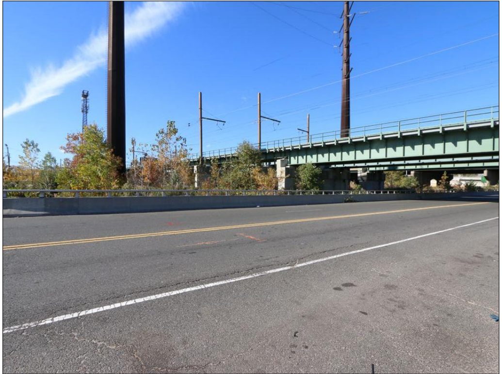
View west of the NEC/PRR Historic District at the southwest end of the APE, where it crosses over County Road and the Jersey City Water Works Historic District (below ground), in the Town of Secaucus.
