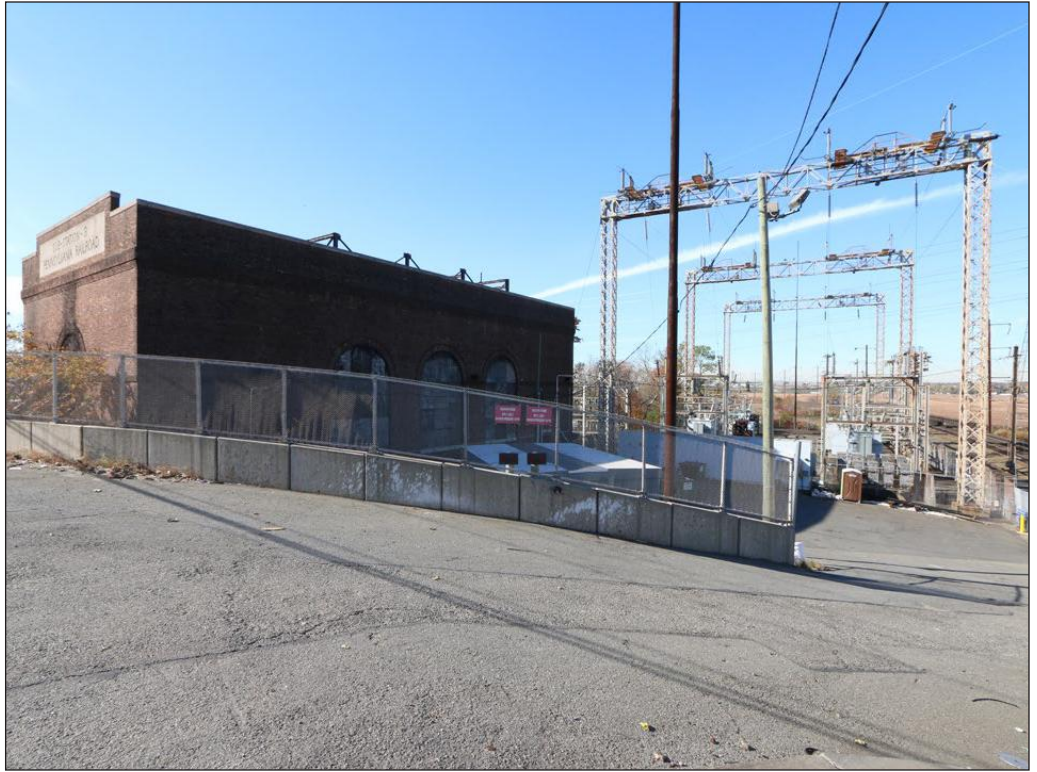
View southwest of the Substation No. 3 building. 7
